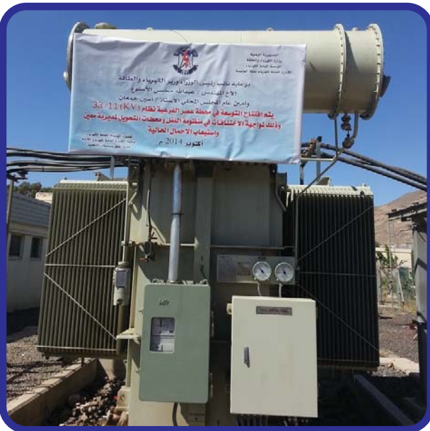
20 MVA Power Transformer with S/S accessories in Asser S/S - Sana'a
