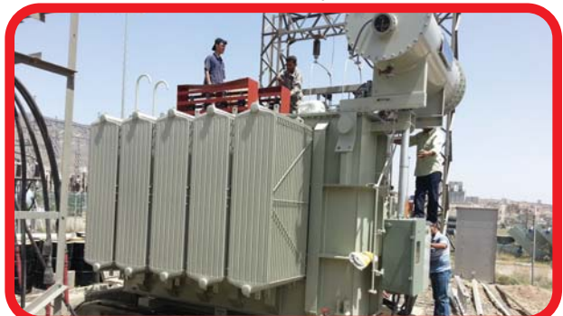
20 MVA Power Transformer with S/S accessories in Qasr Asselah - Shoob - Sana'a
