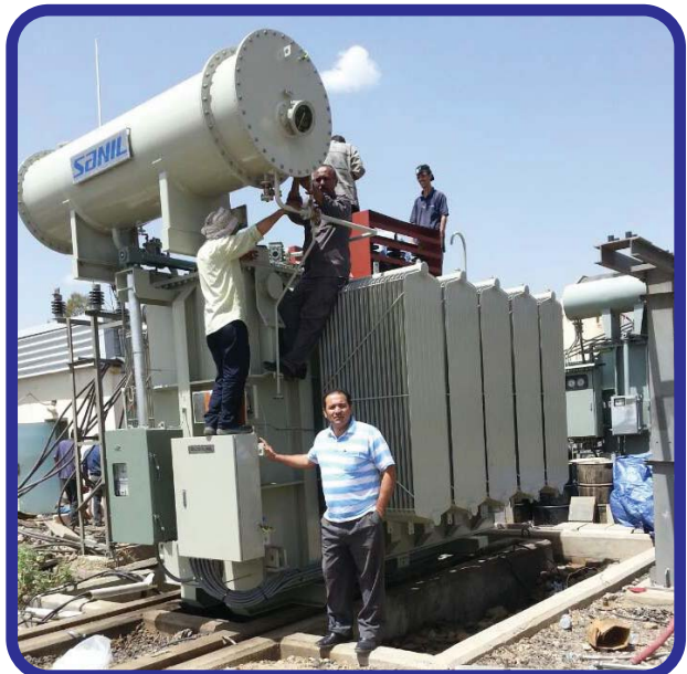
20 MVA Power Transformer with S/S accessories in Asser S/S - Sana'a
