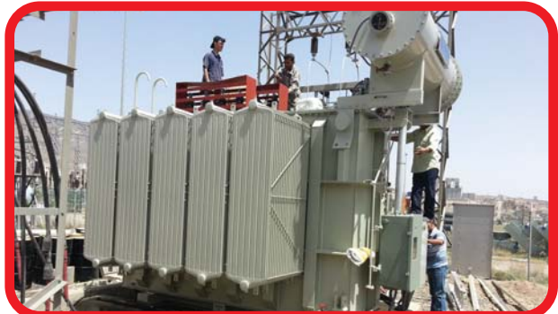
20 MVA Power Transformer with S/S accessories in Qasr Asselah - Shoob - Sana'a
