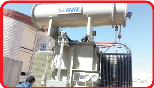
20 MVA Power Transformer with S/S accessories in Qasr Asselah - Shoob - Sana'a
